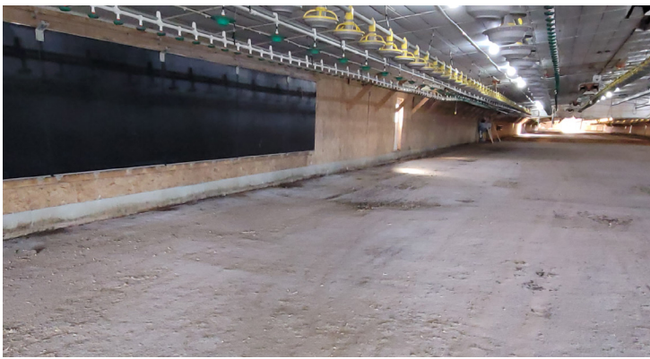
AFTER INSTALLATION AT 1.5 TONS PER 24,000 SQ FT
